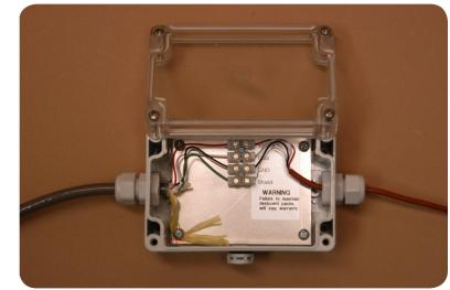
Dry Air Junction Box Wiring
